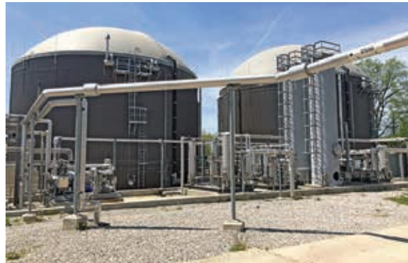
Anaerobic Digester.
